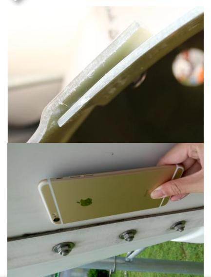
1. Integral moulding, compare with trodictional hand lay-up, whole silo would keep uniform thickness
